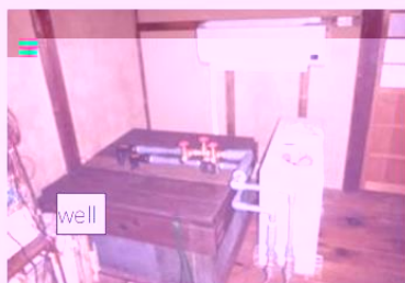
Fig. 3. Well and heat-pump system
